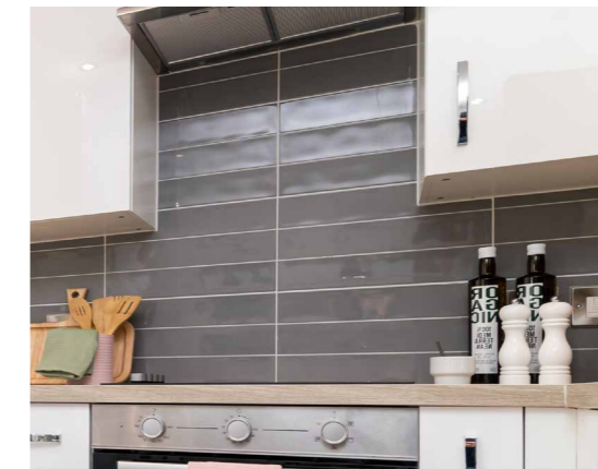
Tiling to underside of cooker hood
